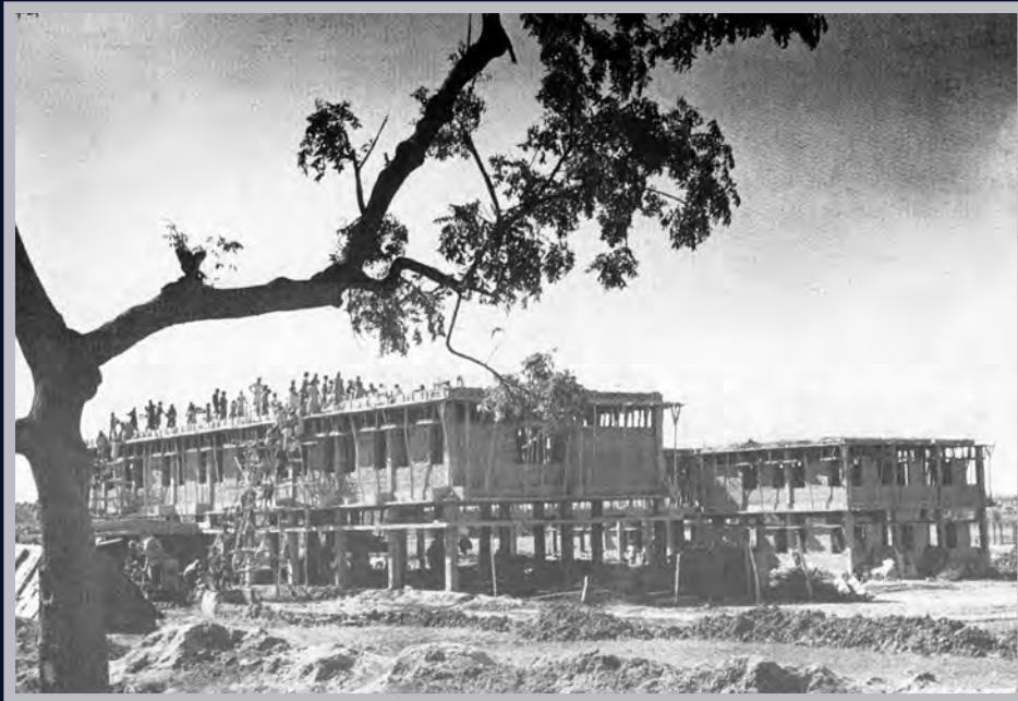
Building complex for the All India Co-ordinated Rice Improvement Project (AICRIP)
