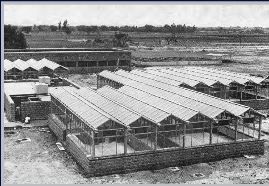
Construction of Glass Houses for Screening Pests & Diseases at AICRIP, Rajendranagar
